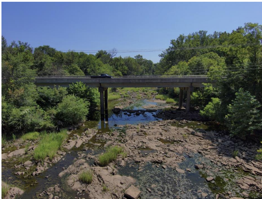
Figure 3.30: Profile View of a Bridge Taken By a UAS.
